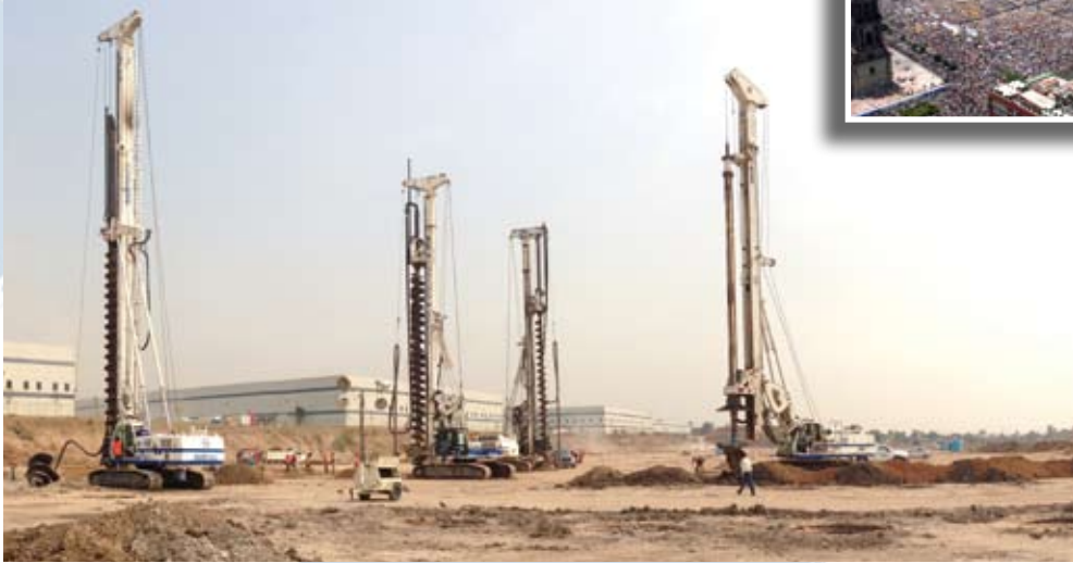
Several Soilmec SF-70 drilling rig for CFA at work in Mexico
