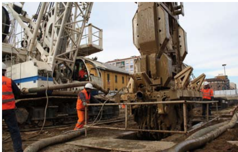
Hydromill positioning into the trench.
