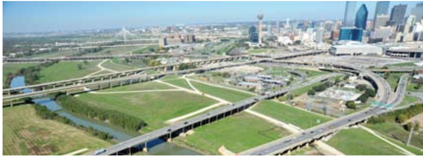
Aerial view of the works for the new bridge.
