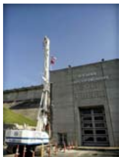
ON COVER Soilmec SR-80 at Wolf Creek Dam.
