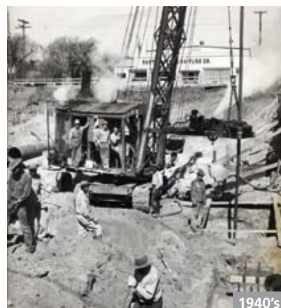
Steam powered drilling rig in one of the first jobsites.
