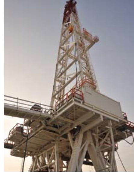
Drillmec rig on its first well in Dharan (KSA).
