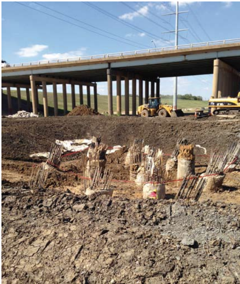
Detail of piles.
